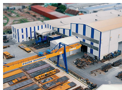
PREIS SEVNICA d.o.o. Steel Construction and Welded Constructions
